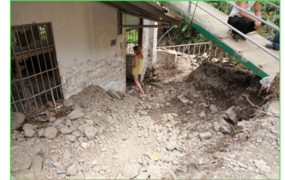
Household affected by a mudslide
