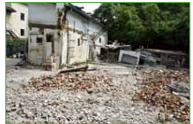
Some of the structures were leveled to the ground.
